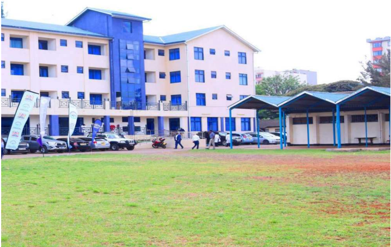
KEWI Water Resource Centre Building
