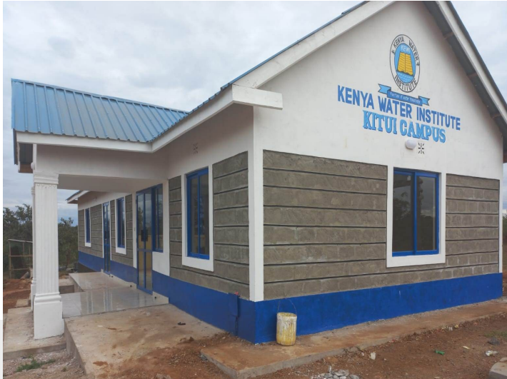
Administration Block that is nearing completion at Kitui Campus.
