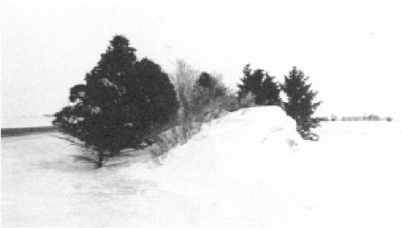
Figure 5.9 Deep drafts at a living snow fence.
