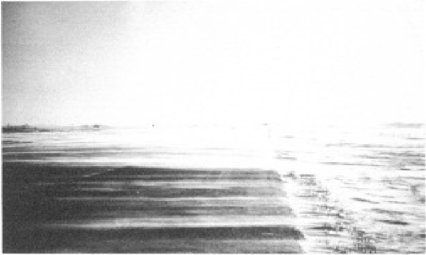
Figure 5.5 Smooth cross-section and flat foreslopes provide drift-free roadway.
