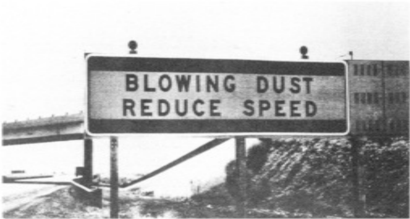
Figure 7.13 Radio-controlled roadside dust-warning sign maintained by Arizona Department of Transportation. Note radio antennae in upper right (after ADOT 1976).
